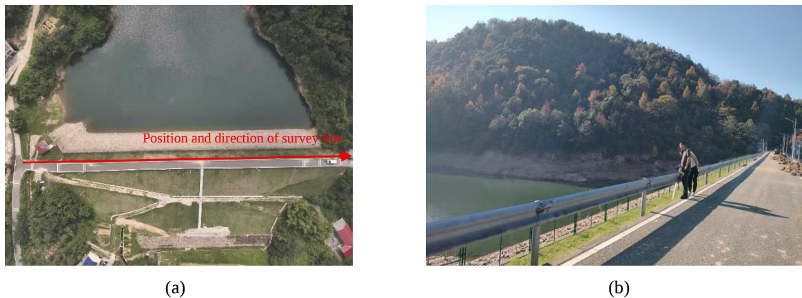
Figure 9. (a) An aerial photograph; (b) a field photograph of Dishuiyan Reservoir
